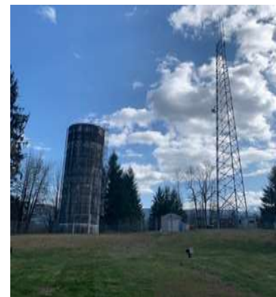
Figure 4-2 Sauk-Suiattle Water Storage Tank and Communications Tower
